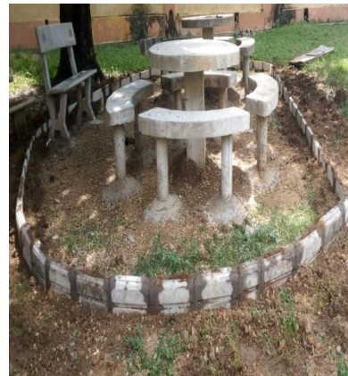
Fig. Installation of kerbs
