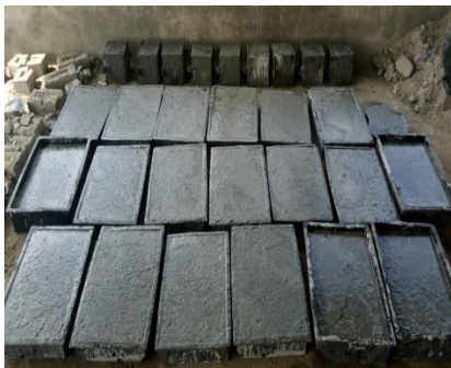
Figure 1: Casting of Kerbs cubes
